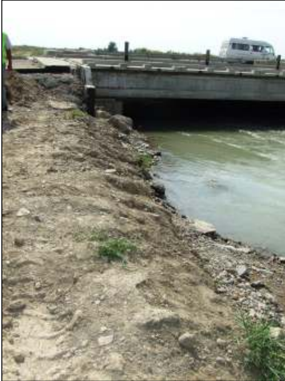
AKM – Lack of sediment and erosion control measures adjacent to waterway
