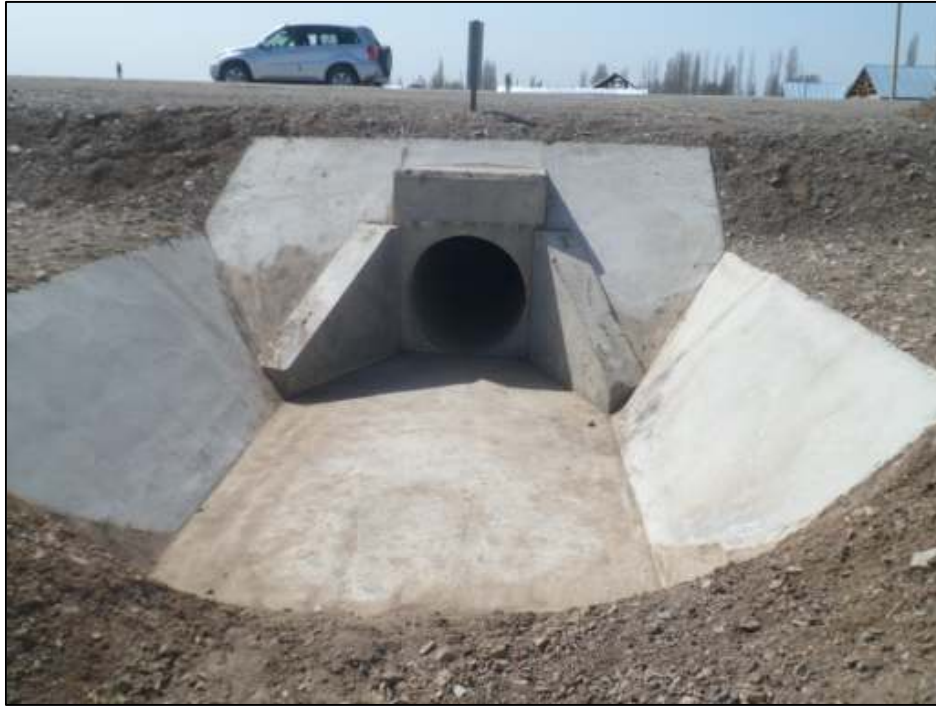
Examples of AKM rehabilitation works – culvert outlet (above) and cattle crossing (below)
