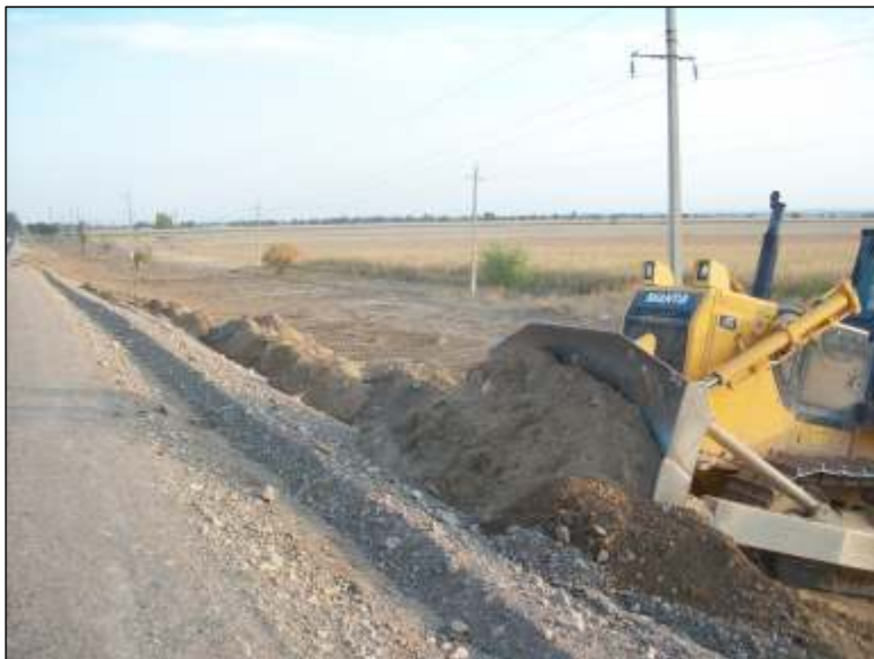
Examples of AKM rehabilitation works – Road shoulder and diversion track rehabilitation works in progress
