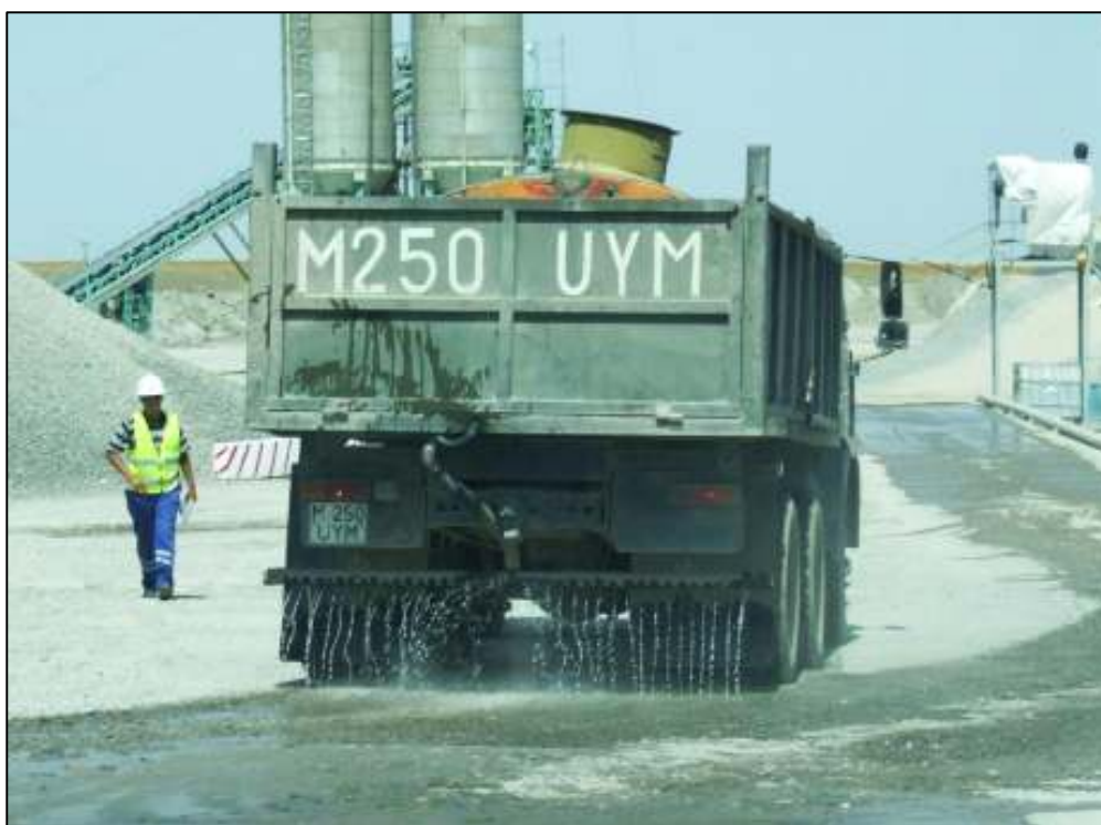
Below – Dust control by water truck at concrete batching plant
