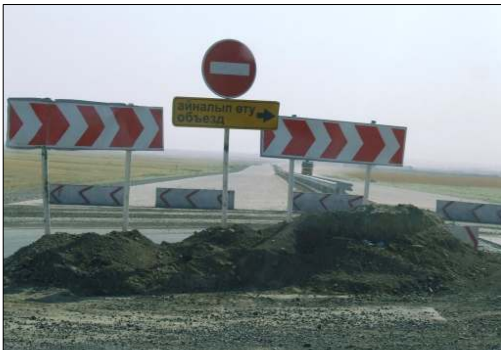
Above – Signs diverting traffic from new carriageway to old highway – contradiction in direction signs
