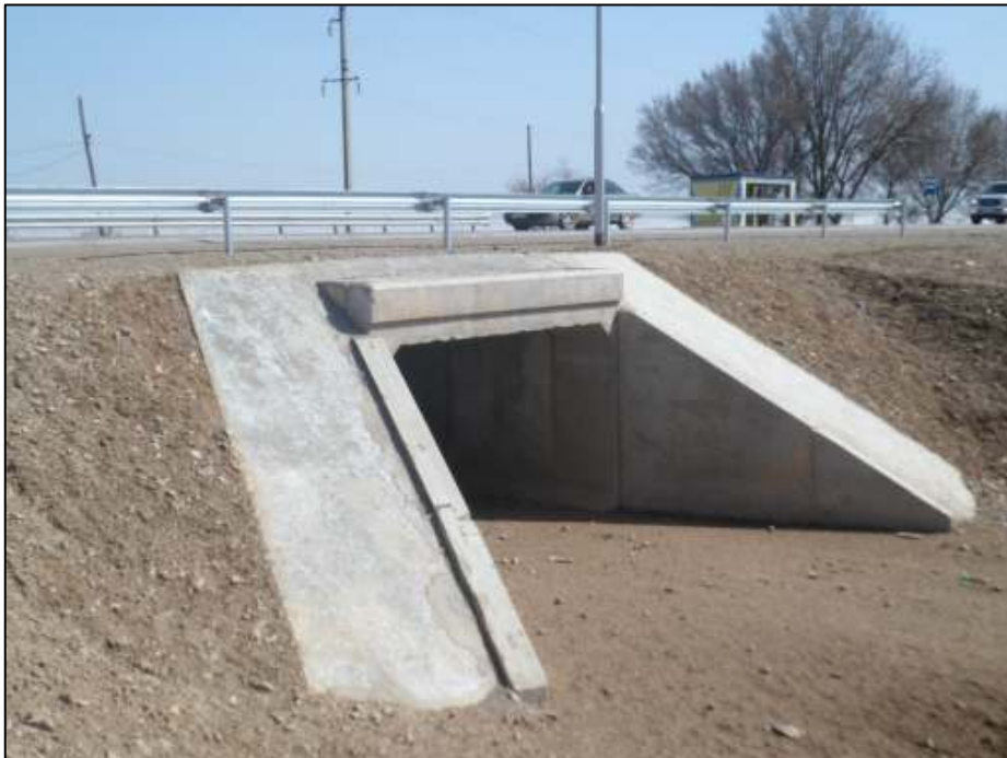
Examples of AKM rehabilitation works – culvert outlet (above) and cattle crossing (below)
