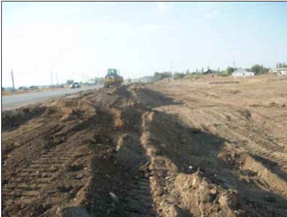
Examples of AKM rehabilitation works – Road shoulder and diversion track rehabilitation works in progress
